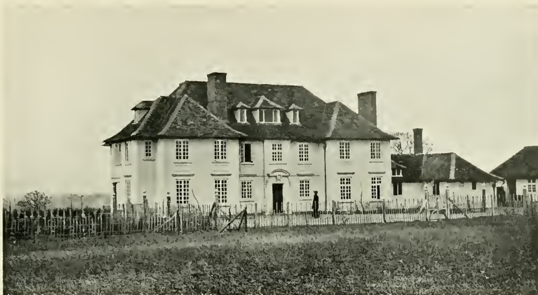
THE ARCHITECT'S OWN RESIDENCE, BREACH HOUSE, CHOLSEY, BERKSHIRE. VIEW OF THE NORTH-WEST OR ENTRANCE FRONT. THE WALLS ARE COVERED WITH SANDED STUCCO WASHED WITH COLOUR, THE ROOFS ARE TILED
